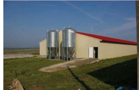
Picture: A 66 x 18.3 Meter steel building in 6 sections with a fat-tener capacity of 6 x 250 pigs—or more than 4,000 pigs / year.
